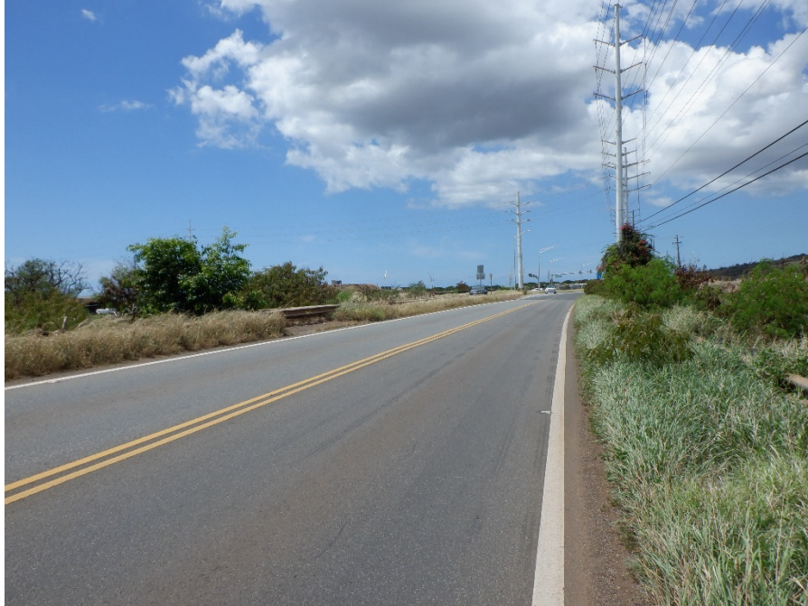
PHOTO 1 EAST APPROACH LOOKING WEST
