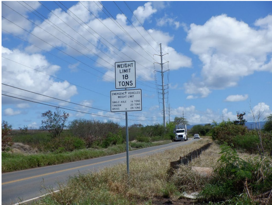
PHOTO 6 LOAD POSTING SIGNS ON FARRINGTON HIGHWAY AT WEST APPROACH TO BRIDGE
